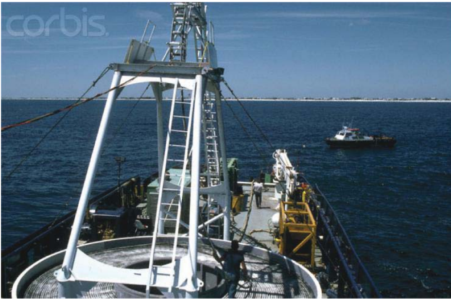
FIGURE 7.14 Laying transatlantic cable.
