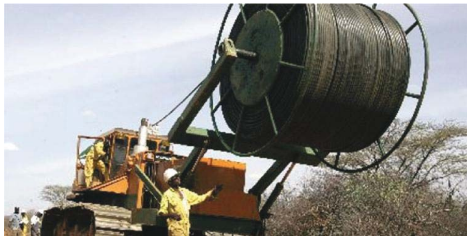
FIGURE 7.13 Laying the cable.
